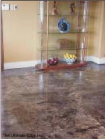
One of the advantages of concrete is its tremendous versatility. Not only can it be colored or stained to match any hue, but you can select your texture, too (To change the texture, see 'overlays' under the Special Applications section of the document).
