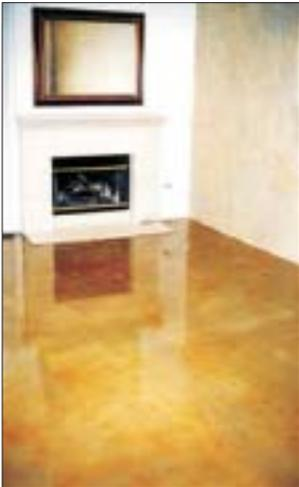
Polishing concrete is similar to sanding wood. Heavy-duty polishing machines equipped with progressively finer grits of diamond-impregnated segments or disks (akin to sandpaper) are used to gradually grind down surfaces to the desired degree of shine and smoothness.
