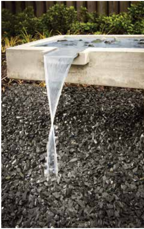
OPPOSITE: THE BENCH WAS MADE IN ONE PIECE USING GLASS-FIBER-REINFORCED CONCRETE. NO PIGMENT OR SPECIAL FINISHES WERE ADDED. ABOVE LEFT TO RIGHT: THE WATERFALL, GENERATED BY A RECIRCULATING PUMP, FLOWS OVER THE EDGE IN A GENTLE CASCADE; A FURROW IN THE BACK OF THE BENCH CHANNELS THE WATER OVER A BED OF NATIVE RIVER ROCK; COMBINING THE ORGANIC ELEMENTS OF CONCRETE, STONE, AND WATER, THIS WABI-SABI STYLE GARDEN BENCH IS THE IDEAL SPOT FOR REFLECTION AND MEDIATION.
