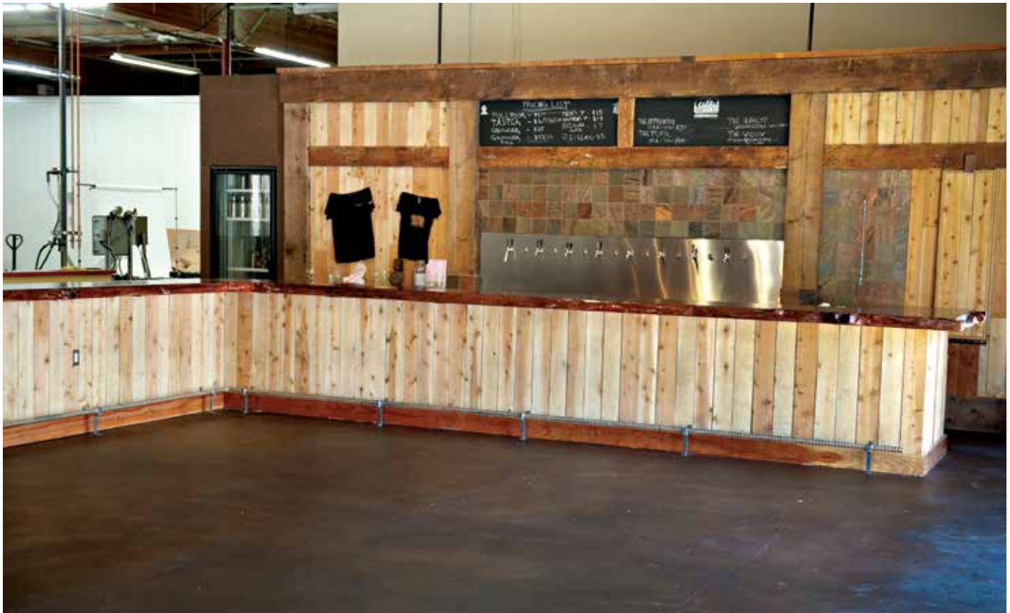
In Societe's tasting room, the floors were acid stained in a warm walnut shade and then protected with a polyurethane sealer.
