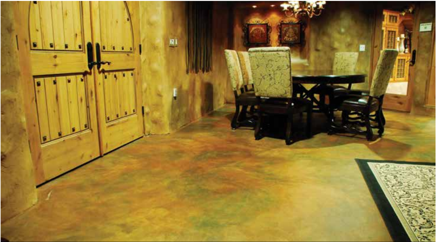
Another example of a tasting room floor treated with a stain. Here two colors of Westcoat water-based stain were used for a mottled look, followed by sealing with a clear epoxy and satin polyurethane.
