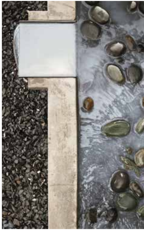
OPPOSITE: THE BENCH WAS MADE IN ONE PIECE USING GLASS-FIBER-REINFORCED CONCRETE. NO PIGMENT OR SPECIAL FINISHES WERE ADDED. ABOVE LEFT TO RIGHT: THE WATERFALL, GENERATED BY A RECIRCULATING PUMP, FLOWS OVER THE EDGE IN A GENTLE CASCADE; A FURROW IN THE BACK OF THE BENCH CHANNELS THE WATER OVER A BED OF NATIVE RIVER ROCK; COMBINING THE ORGANIC ELEMENTS OF CONCRETE, STONE, AND WATER, THIS WABI-SABI STYLE GARDEN BENCH IS THE IDEAL SPOT FOR REFLECTION AND MEDIATION.
