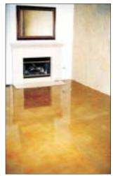
Polishing concrete is similar to sanding wood. Heavy-duty polishing machines equipped with progressively finer grits of diamond-impregnated segments or disks (akin to sandpaper) are used to gradually grind down surfaces to the desired degree of shine and smoothness.
