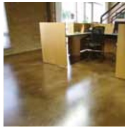
LIFE DECK COATING INSTALLATIONS
