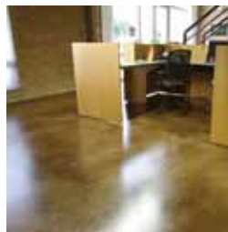
LIFE DECK COATING INSTALLATIONS
