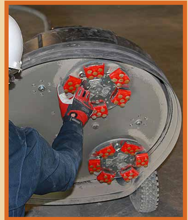
CONCRETE POLISHING & SEALING
