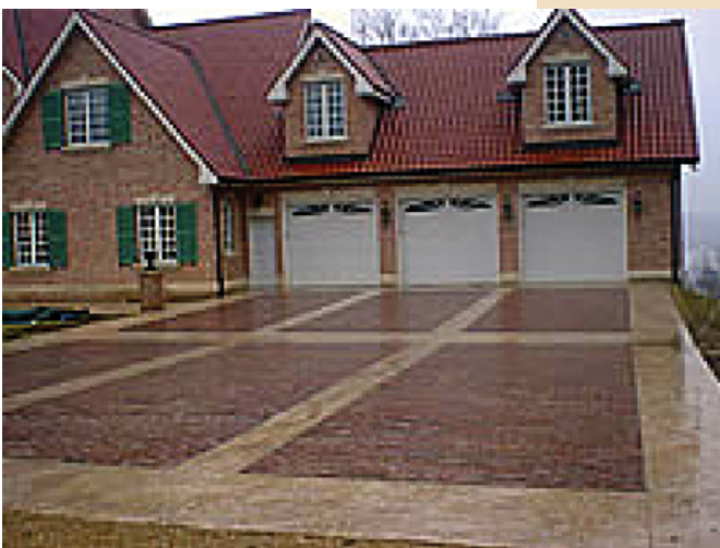
D&D SUPERIOR CONCRETE CONSTRUCTION
