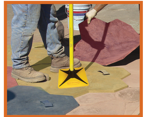
Stamping tools should look and feel sturdy with thick handles and crisp, clean textures.
